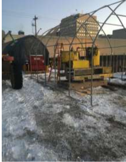
Grouting machine within the temporary shelter.
