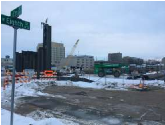
Friday morning progress of sheet piling along Elm Street.
