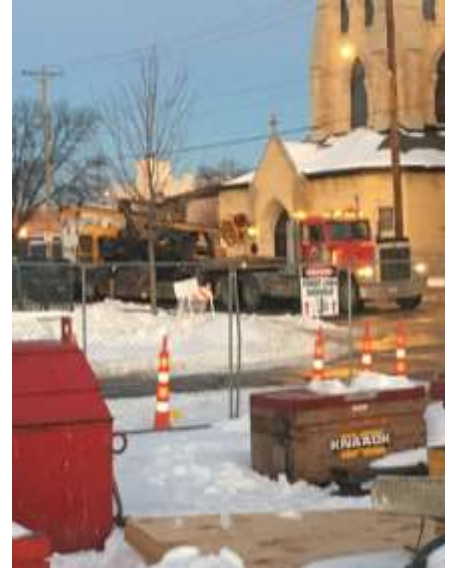
Delivery of the second tieback auger machine.
