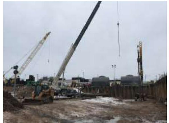
A smaller crane that was delivered on Friday will be used to hoist tieback rods into the augured holes.
