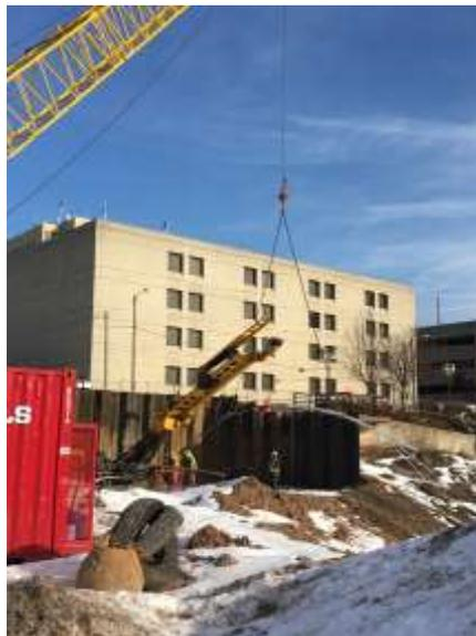
A crane was utilized to hoist the tieback rods into place while another crew member fed it into the augured hole.
