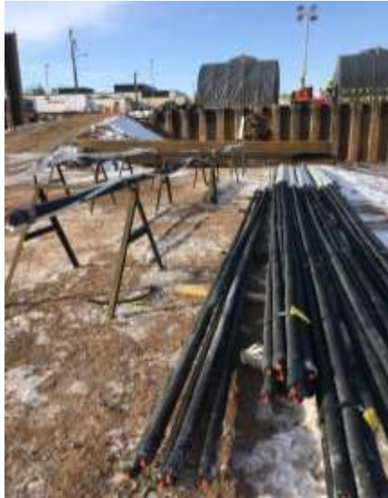
Tieback rods being prepped for installation. PVC tubes around the rod are for grouting the exterior of the rod. The grout is what creates the resistance to keep the rod in place once installed.
