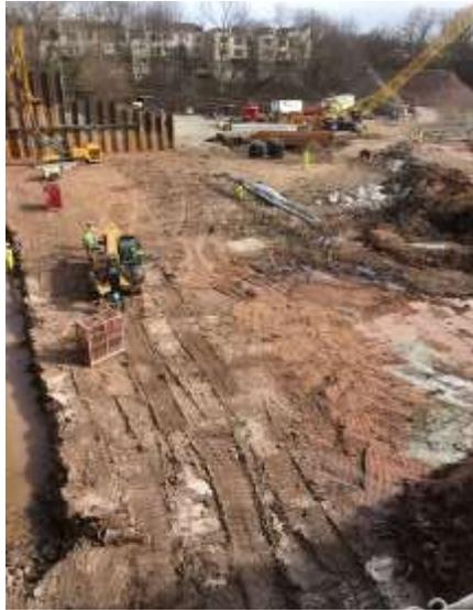
The extent of the mass excavation of Tier 3. Michels can also be seen prepping work for tieback installations along Lawrence Street.
