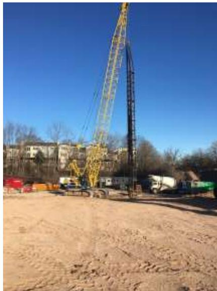
Michels' diesel hammer being utilized to drive the test pipe pile into the ground.
