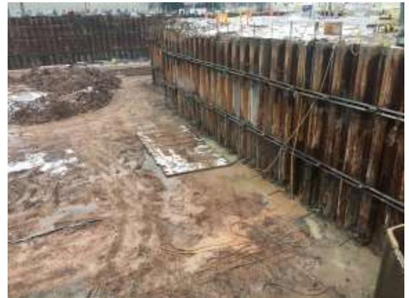
View of the Elm Street side of the project. The majority of the tieback anchors are installed, except for a few that will require a duplex auger to cut through the old foundations buried in the soils.
