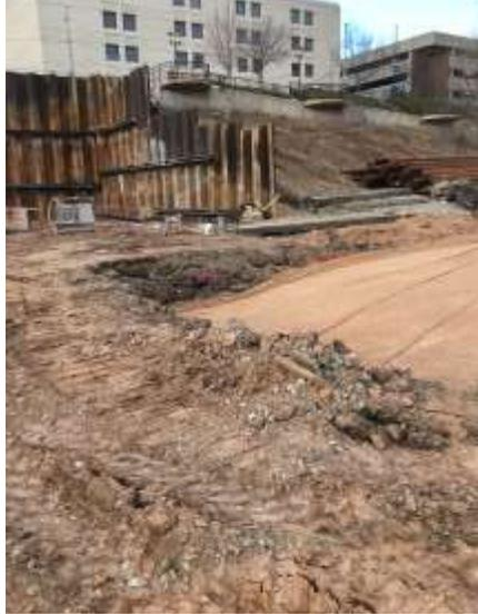
Location of the large existing footing; it was removed and backfilled to allow the pipe piling to be installed.
