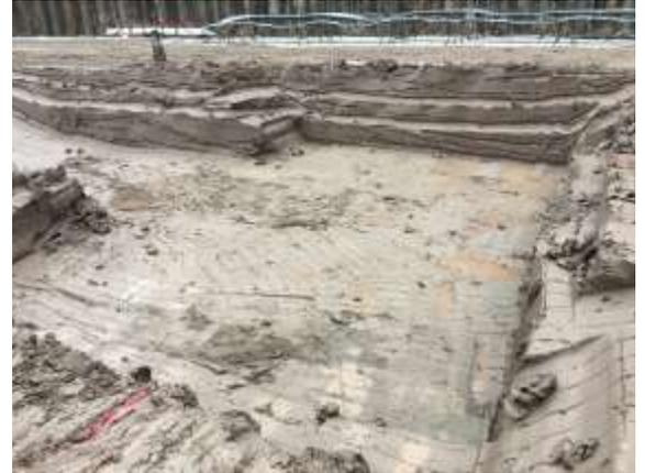
Location of the future freight elevator. This was dug out to allow access for the drill rig coming Monday morning to drill the hole for the hydraulic lift of the elevator.
