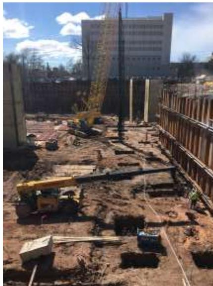
As Miron pours concrete along Lawrence Street, Michels continues testing tieback anchors and installing pipe piling along Elm Street.
