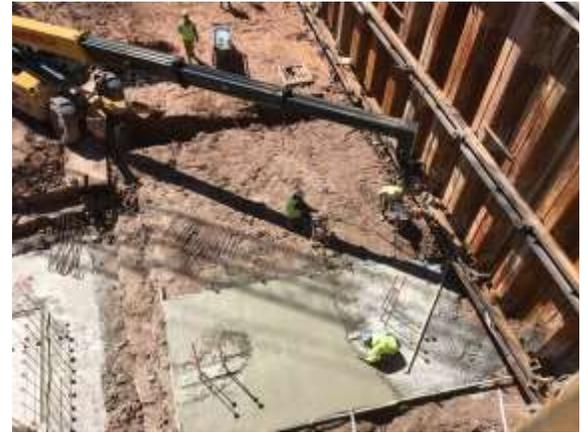
Concrete finishers completing a pile cap in the northwest corner of the site.
