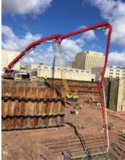
Miron's pump truck pouring concrete into the freight elevator pile cap early in the week.
