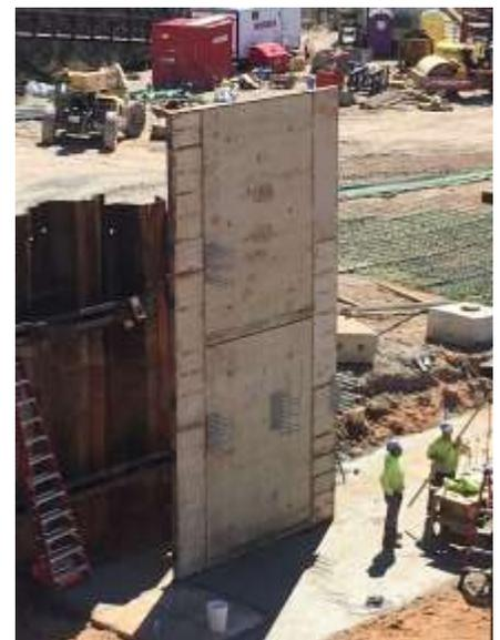
Miron setting the first form for the east wall. Notice the embedded plates anchored to the forms. These will be used to attach rods from the concrete walls to the sheet piling, ensuring that the building will not shift over time.
