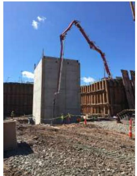
Crews working on the interior grade beams and pile caps with the finished freight elevator shaft in the background.
