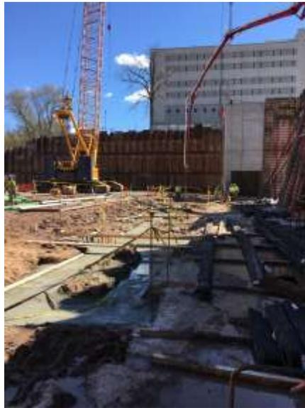
Concrete being poured into the pile caps and grade beams for the interior walls of the exhibition hall.
