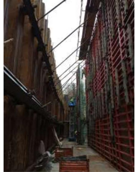
This area is in between the sheet piling and the exterior of the concrete walls. A thinner concrete mat was poured in this area to provide easy mobility for the crews.
