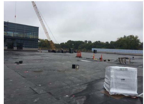
Waterproofing of the plaza deck continues.
