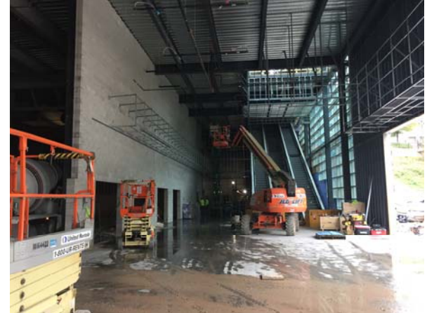
Pre-function area: the full-height CMU wall is complete. MEP installation continues.
